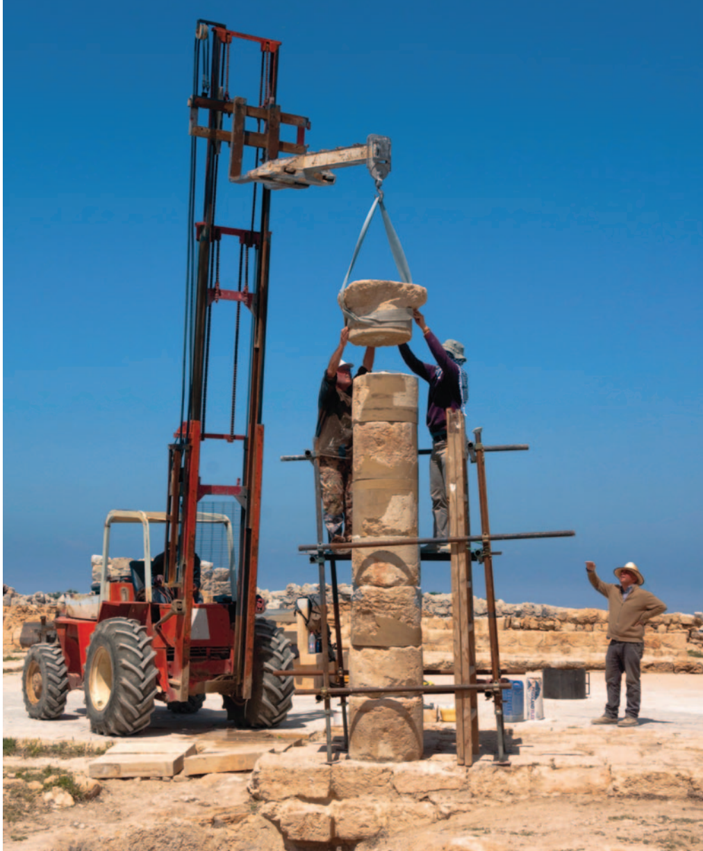
FIGURE 51: Ueli Bellwald and Tamás Dobrosi superimpose the Doric capital while the author (on the right) directs Khader Apsi on the crane in maneuvering the lifting. Behind the camera, Tamás Dósa Papp; view from the east.
