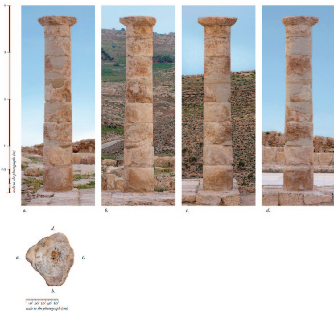
FIGURE 53: The photographic profiles of the re-erected Doric column, as viewed from northeast (a), northwest (b), southwest (c), southeast (d), and from above (on the left, the abacus). The five shots were taken with a telephoto lens, from a great distance, to avoid the distorted perspective of a wide-angle lens. We consider the two columns not only as architectural and decorative elements of the former royal building-complex but also as restored, colossus-size Herodian objects of art.
