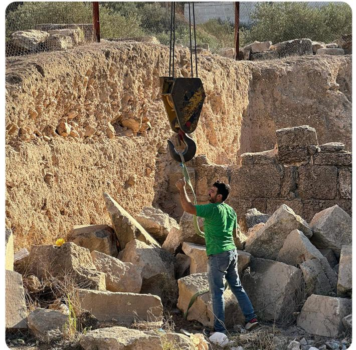
*A worker signals approval to a crane operator, directing the precise placement of an ashlar during stone sorting in front of the stage area of the Capitolias Theater. (Photo by M. Vincent.)*
