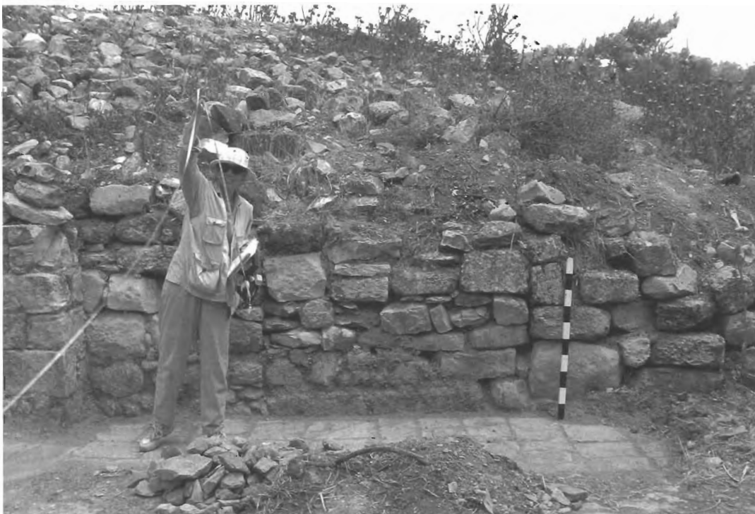
Architectural phasing of the Hubras mosques: There is structural evidence in the Hubras mosque for many building phases. A doorway in the Mamluk extension of the mosque’s northern wall is visible in the background, behind Ellen Kenney
