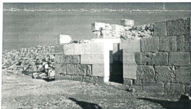
The north side of the tower after restoration. The new stones are the same limestone as the ancient ones. They will weather from white to soft pink in about 10 years.
