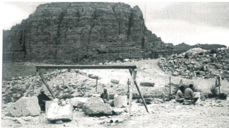
Masons cutting replacement drums for the canopy columns of the Petra Church baptistery
